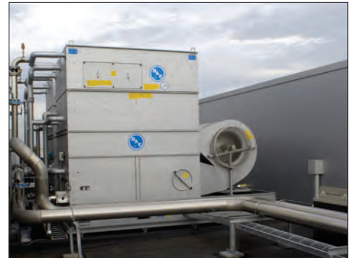
Standard Construction Installation
