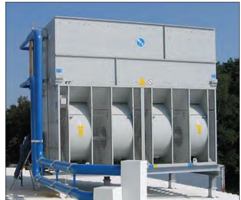
Thermosetting Hybrid Polymer Installation
