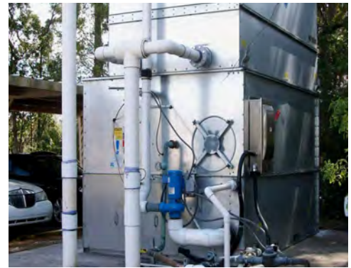
Standard Spray Water Pump
