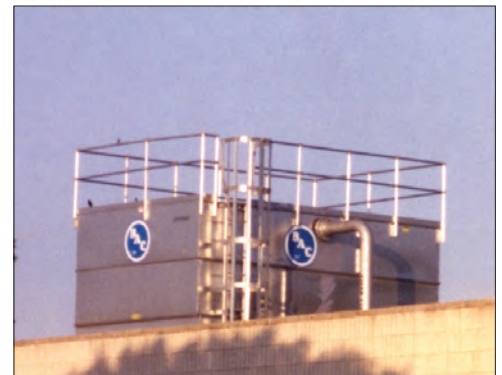
Ladder and Handrail Package
