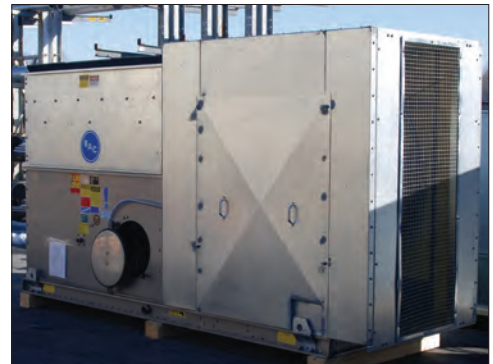
Intake Sound Attenuation
