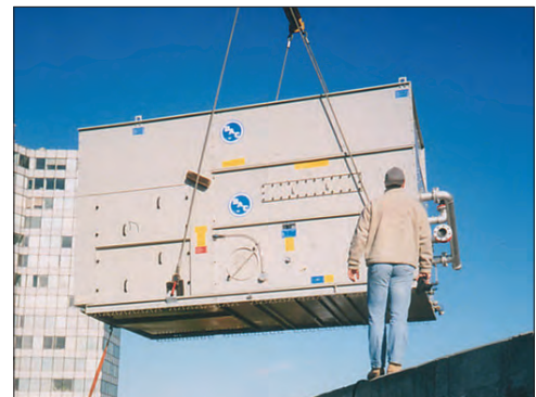
Single Piece Lift of a VFL
