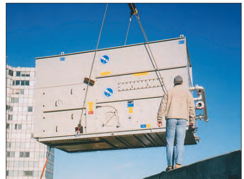
Single Piece Lift of a VFL
